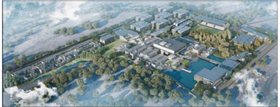
The perspective view of proposed campus of Maharashtra National Law University at Waranga.
